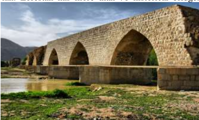
Kashkan Bridge up for renovation
